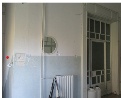
S stena s sondama S33 in S34.
