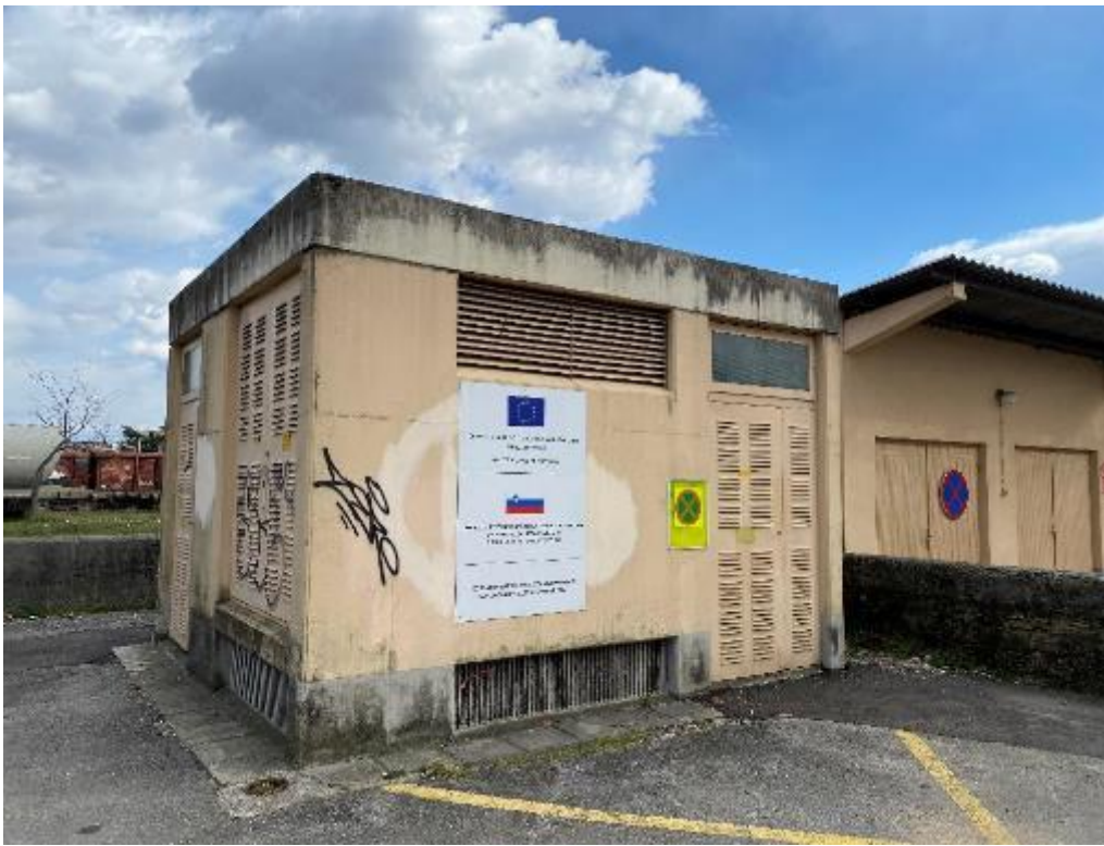
Figure 7: Building at railway "A" 1
