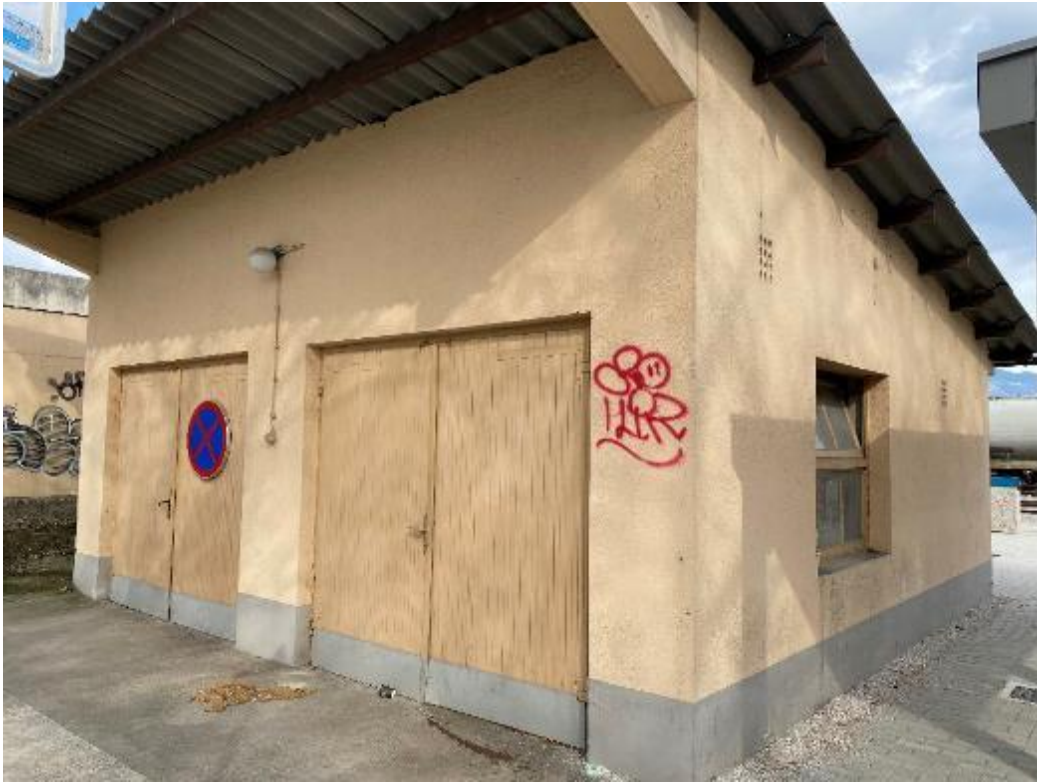
Figure 11: Building at railway "B" 2
