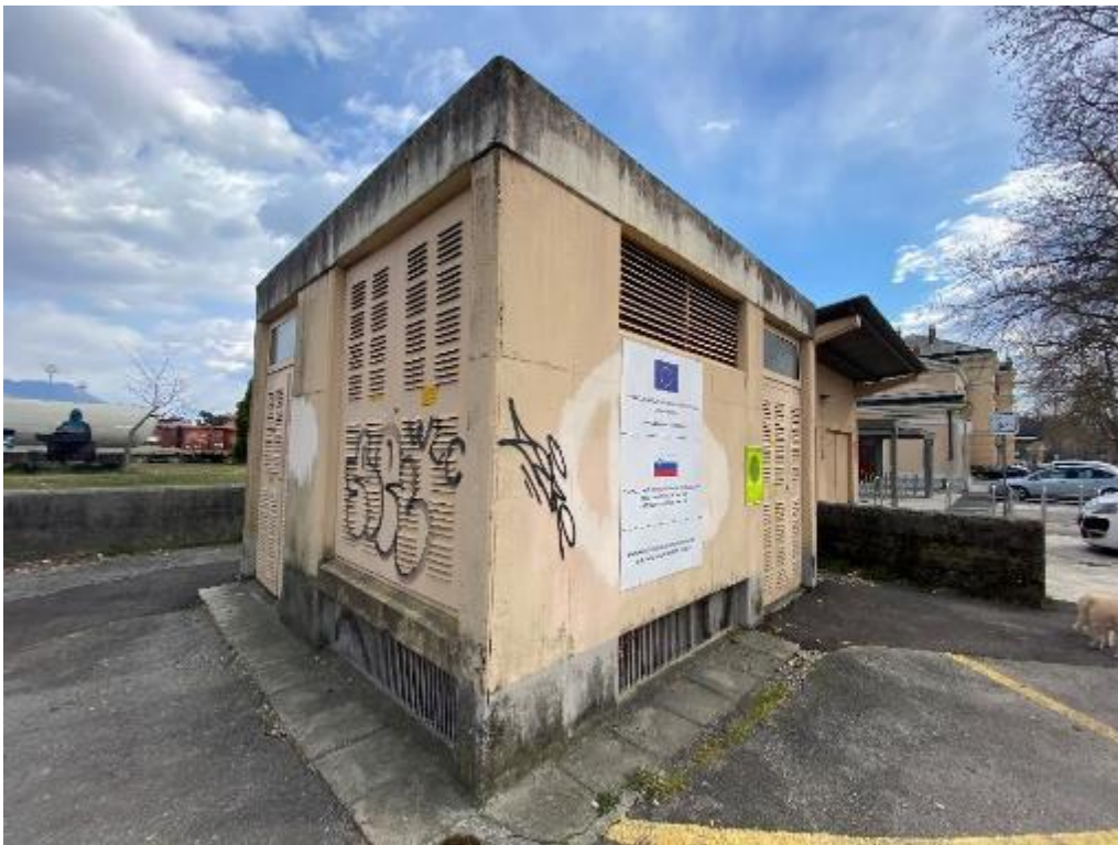
Figure 8: Building at railway "A" 2
