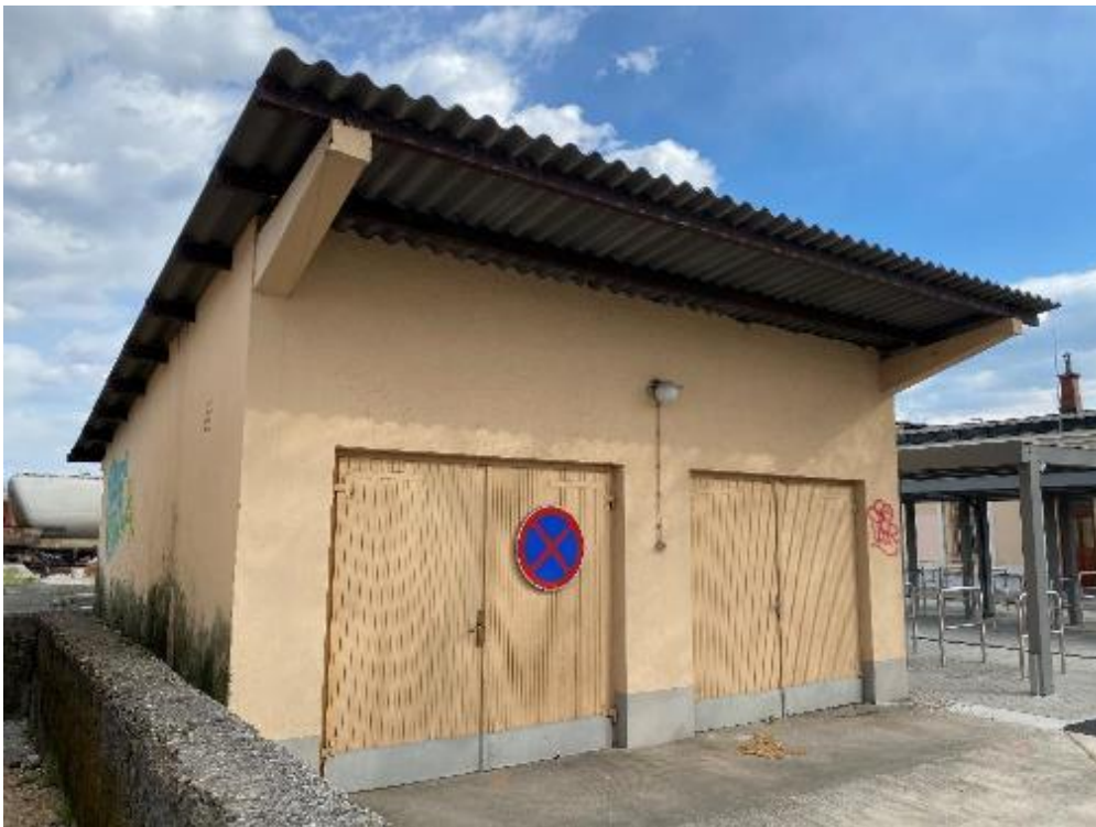
Figure 10: Building at railway "B" 1
